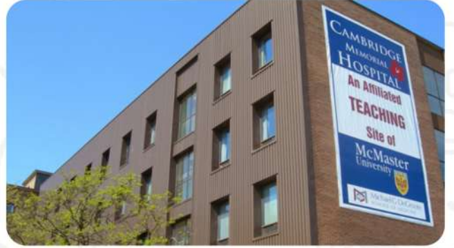
Cambridge Memorial Hospital / Kanada
