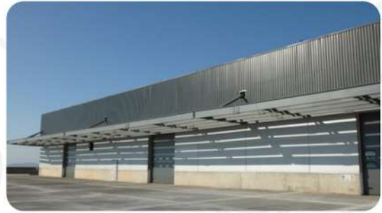
Johnson Control / KOCAELİ
